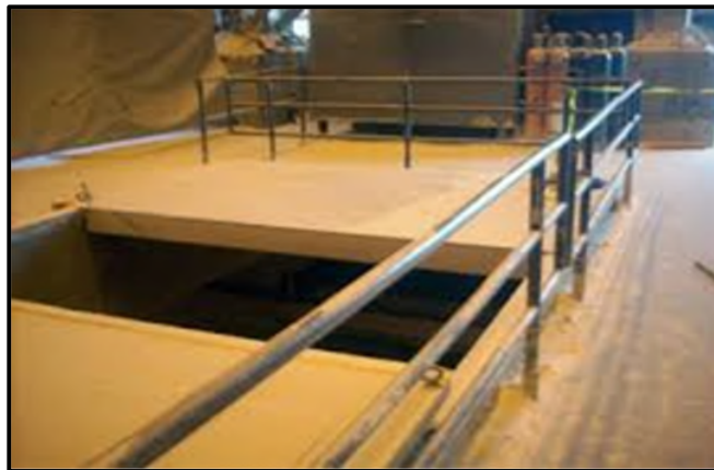
Figure 3: Guardrails around Floor Penetration
