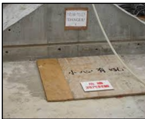
Figure 1: Typical Hole Cover Example
